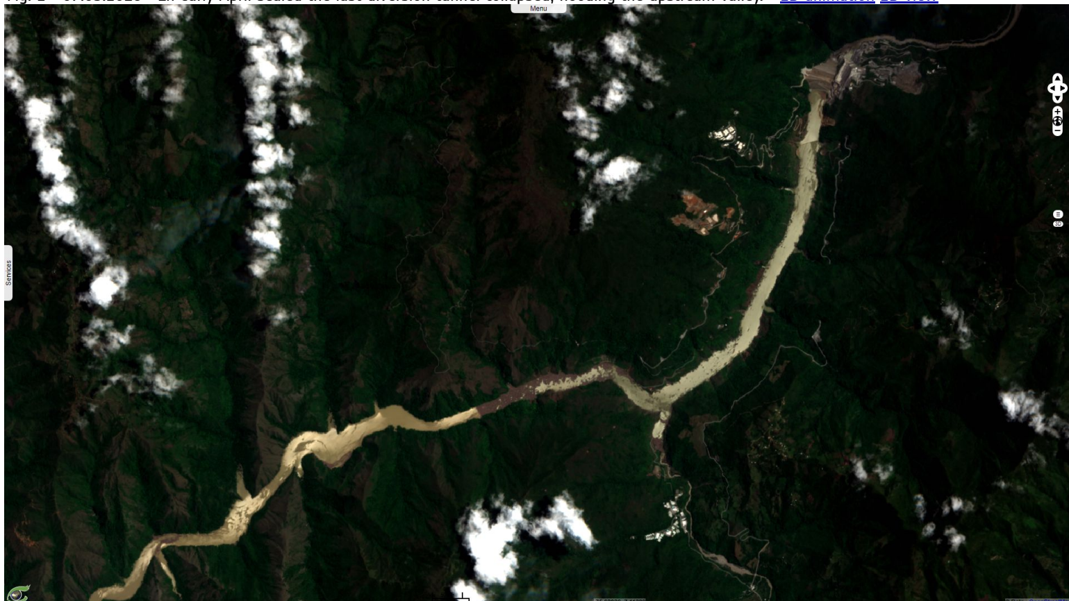
Fig. 2 - 07.05.2018 - In early April sealed the last diversion tunnel collapsed, flooding the upstream valley. - 2D animation 2D view
