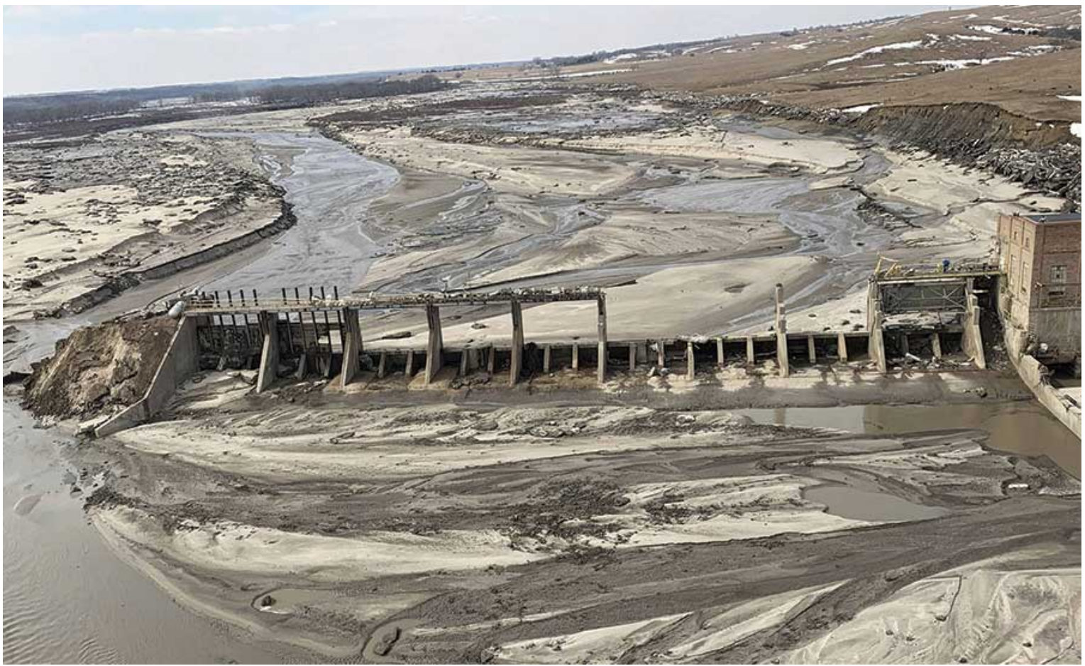
In the midst of historic flooding, truck-sized ice chunks destroyed the Spencer Dam and Bridge, and also took out a campground and house downstream - Source: Engineering News Record .
