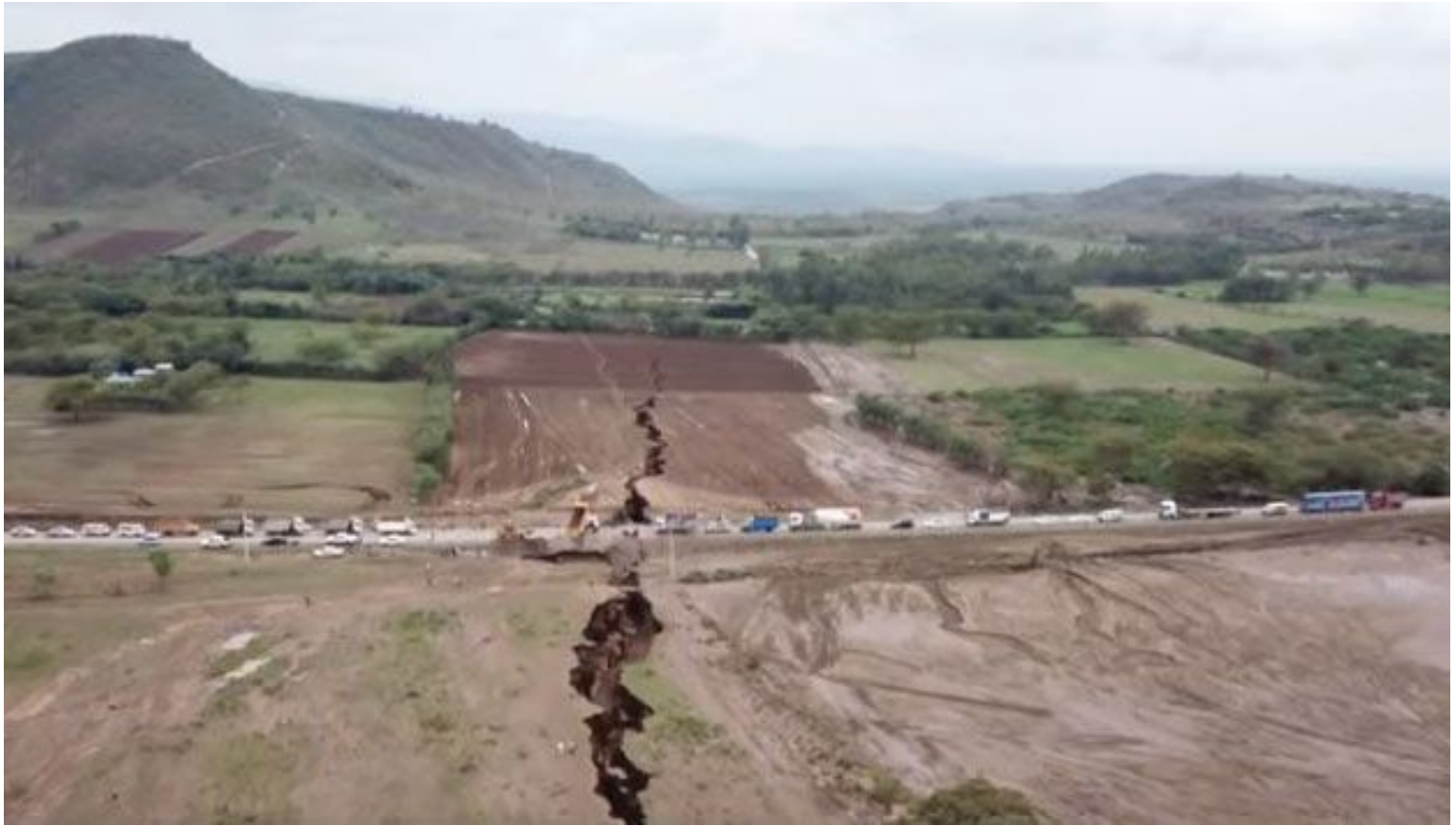
Spectacular 'fissure' that formed on March 19, 2018 (location in fig. 1 & fig. 9) - source : Robert Gichira for Kenyan Nation TV
