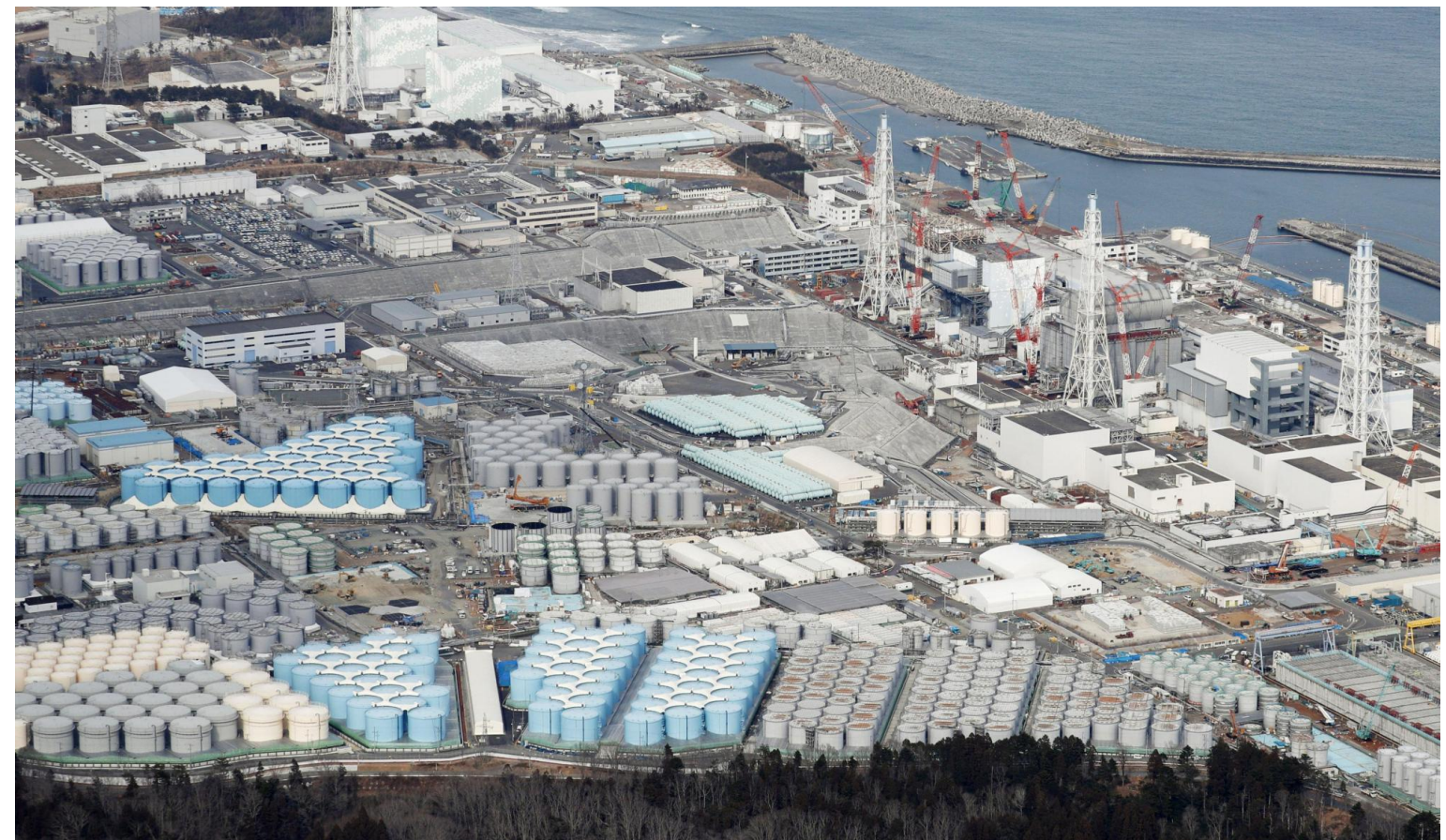
A massive number of tanks storing treated water at the Fukushima No. 1 plant are seen in February - Source: The Japan Times .
